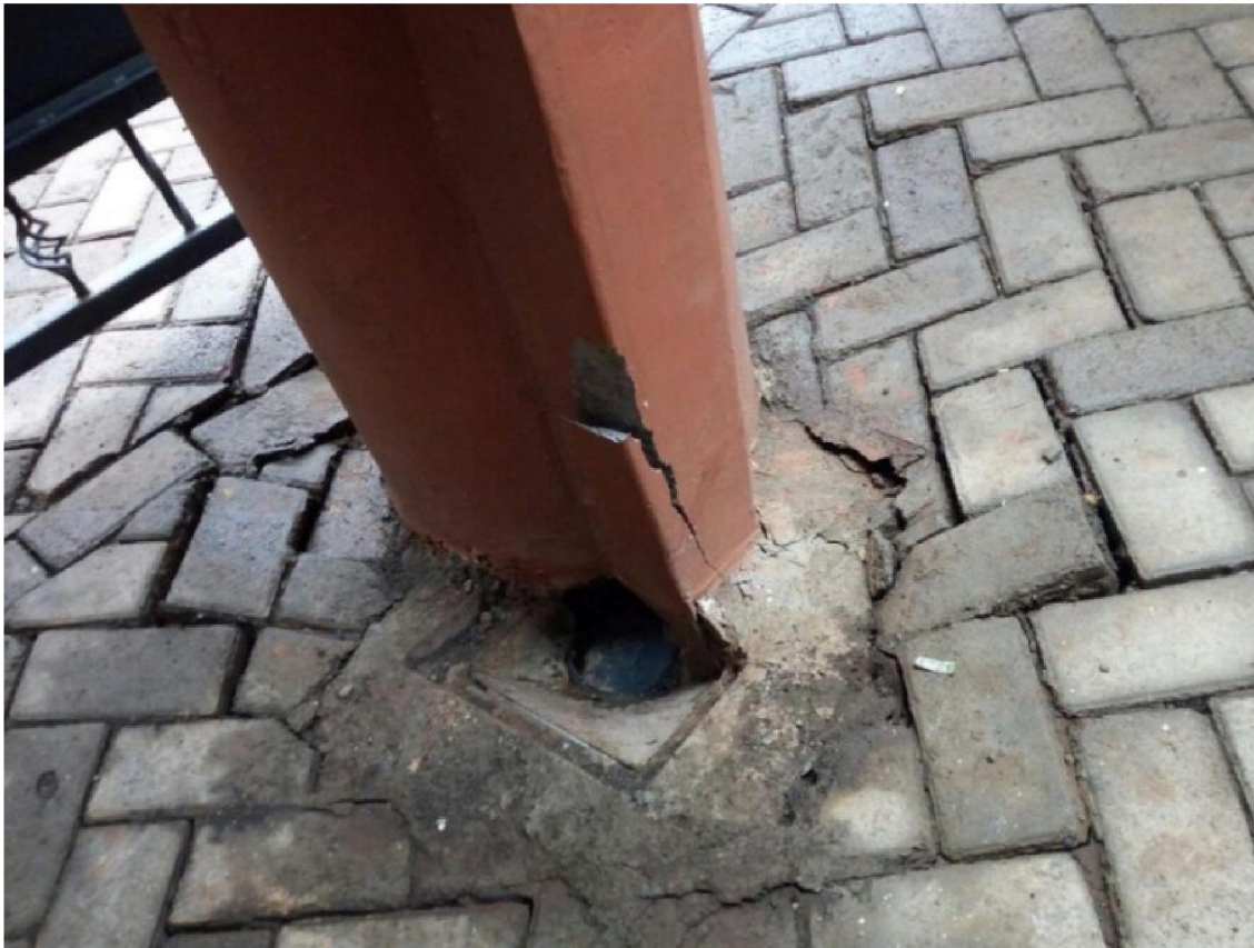
Residents have been asked to vacate a five-storey building in Ruaka after it started showing signs of sinking, November 24, 2016. /COURTESY
