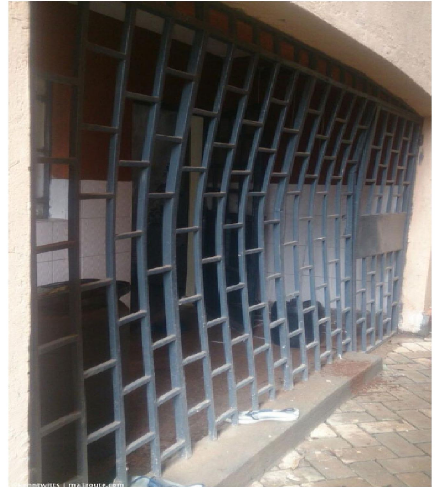
Bent metal grills on the building. PHOTO / COURTESY
